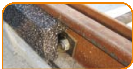
6.3. figure: Vibration insulation of a tram track (Budapest, Kossuth tér)
