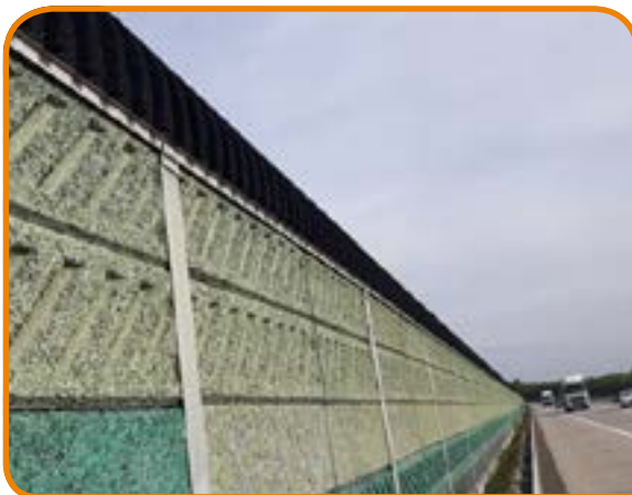
6.2. figure: Increasing the effectiveness of noise barriers – noise barrier tube (M0 Highway)
